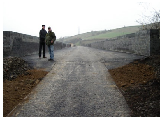
Finished surfacing, rebuilt parapet on right
